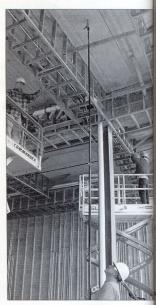
The Viper screws solidly onto a pole for high reach and secure operation for ceiling applications.
