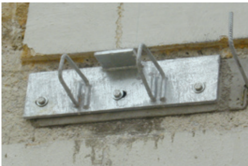
Main upgrading project using Spit Triga Z for bracket of SAI
